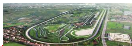
Dongfeng CV Testing ground
