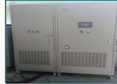
Battery pack charge and discharge test
